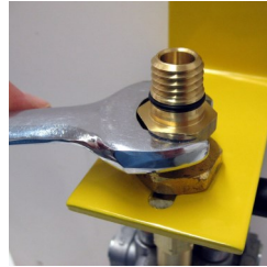
3. Screw the preset MEMO fitting into system inlet.
