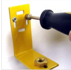
2. Install mounting bracket in an easy access location.
