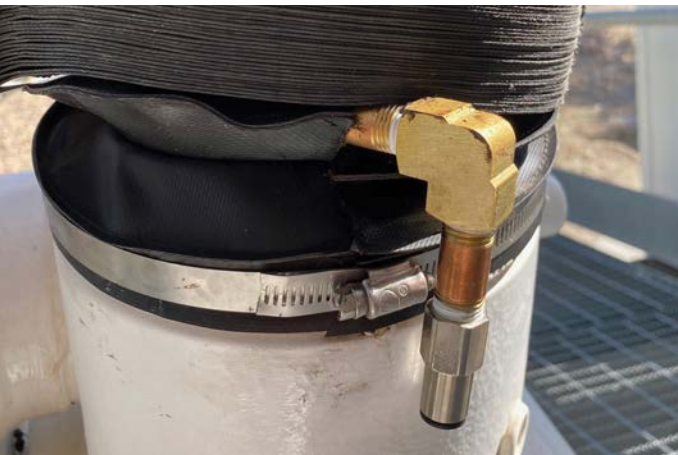
Special piping assembly to reach under the protective boot.
