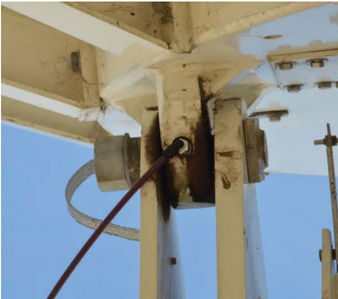
Lubricant line providing grease to a pivot pin.
